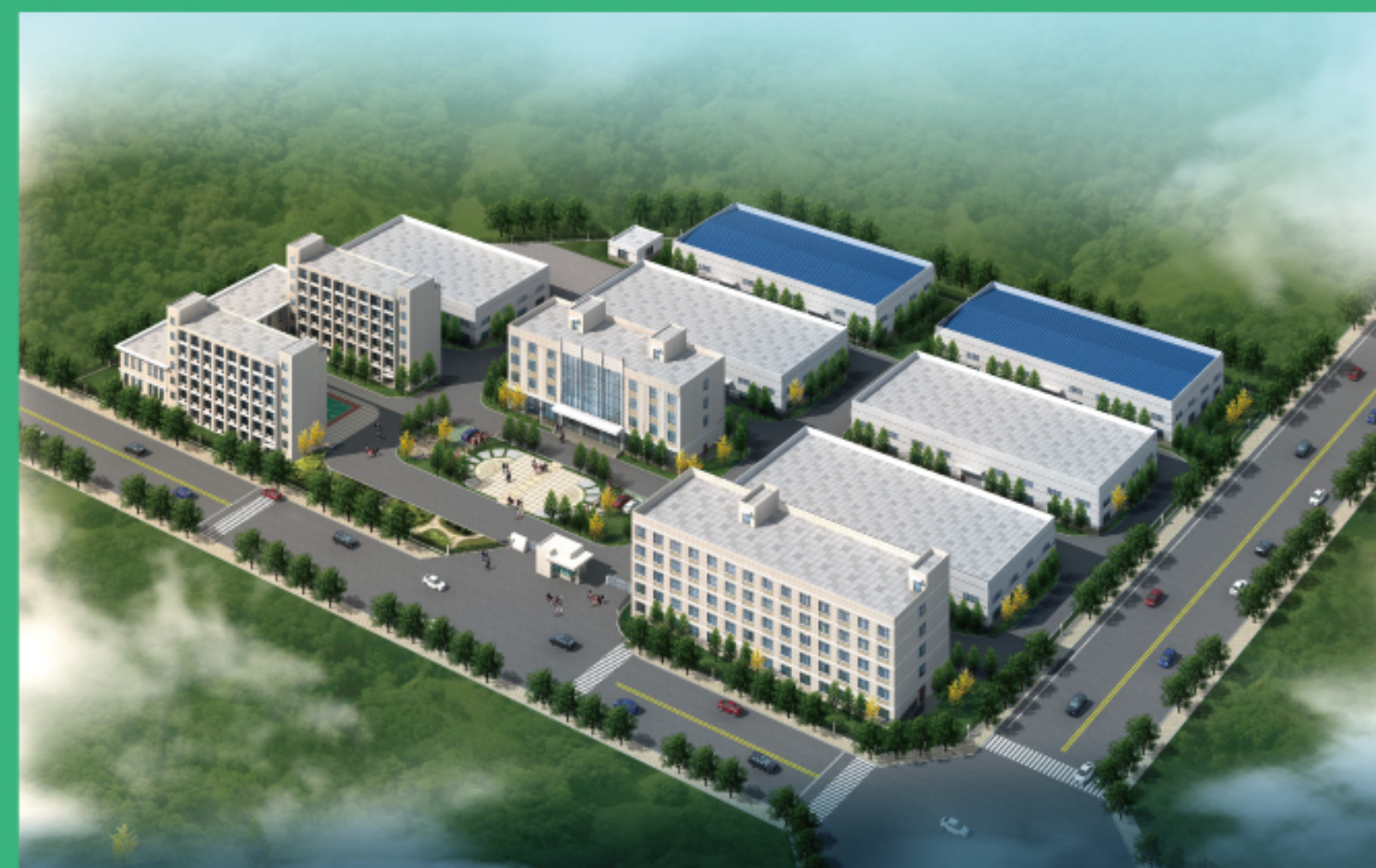
久力工业园鸟瞰图/JULY INDUSTRIAL PARK AERIAL VIEW
