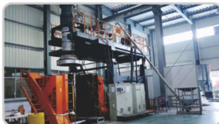
液压机橡胶制品车间 Hydraulic Press Machine
